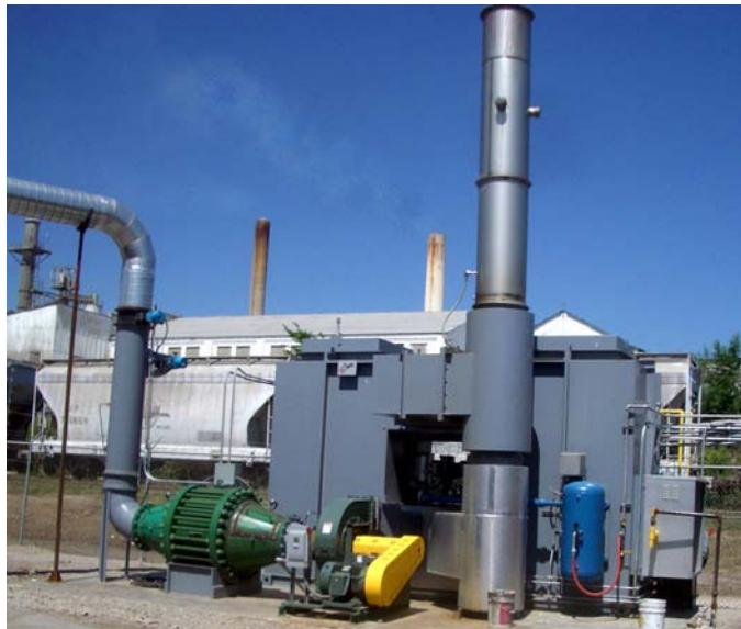
Fig. 7 Systech RTO with waste gas duct from Container Processing Building at left.
