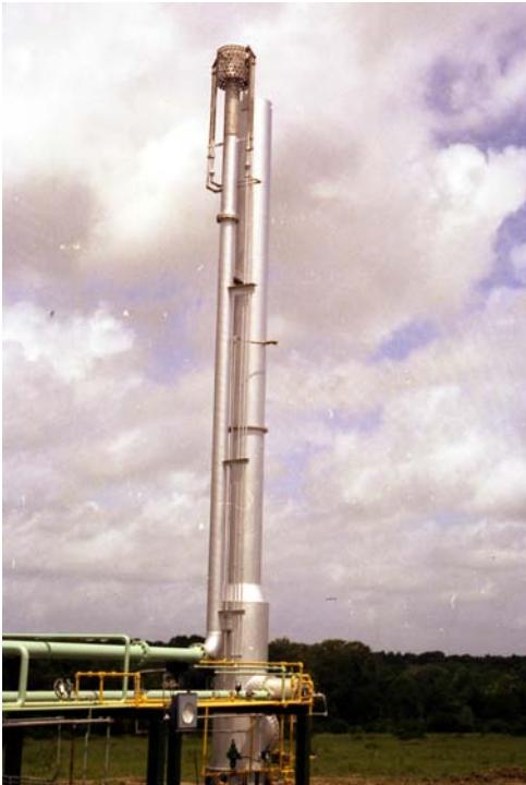
Fig. 3. Elevated Flare supported by an adjacent stack.
