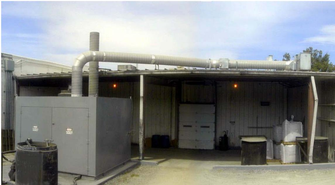
Fig. 1. Systech Container Processing Building vent system – transfer fan on roof feeds activated carbon adsorber at left (grey box with double doors)
