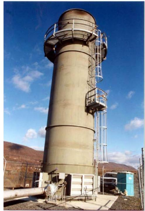
Fig. 4. Typical Enclosed Flare (Courtesy TCE – Ref. 3)
